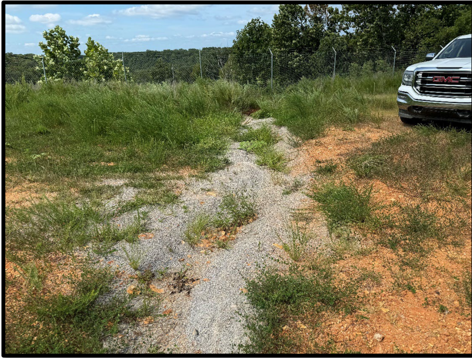
Photograph 17: View of washout present in road between LCS-4 and LCS-5.
