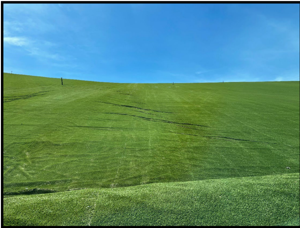
Photograph 6: View of rills present in closure turf of north side of Area 1-2.
