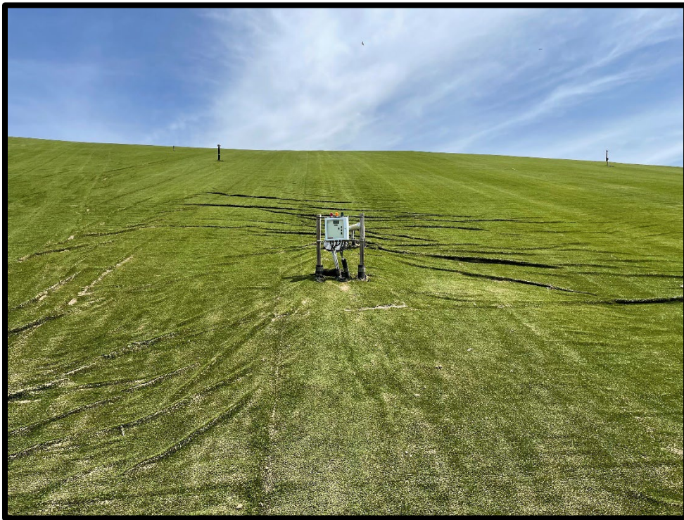
Photograph 10: View of rills present in closure turf near LCS-3.
