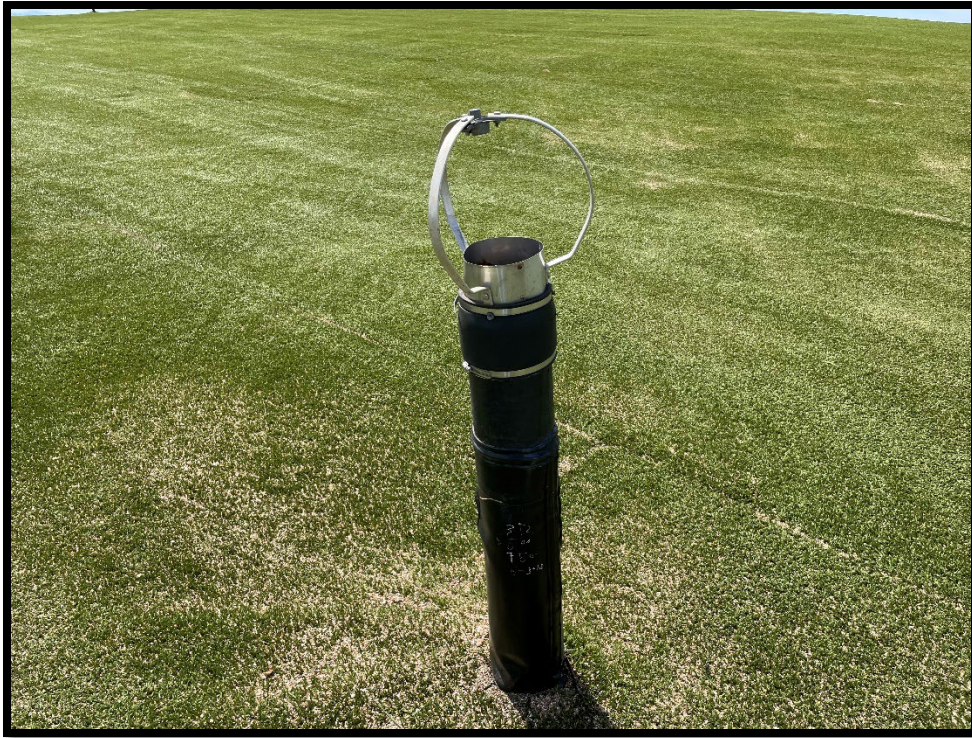
Photograph 3: View of detached turbine vent near LCS-6.
