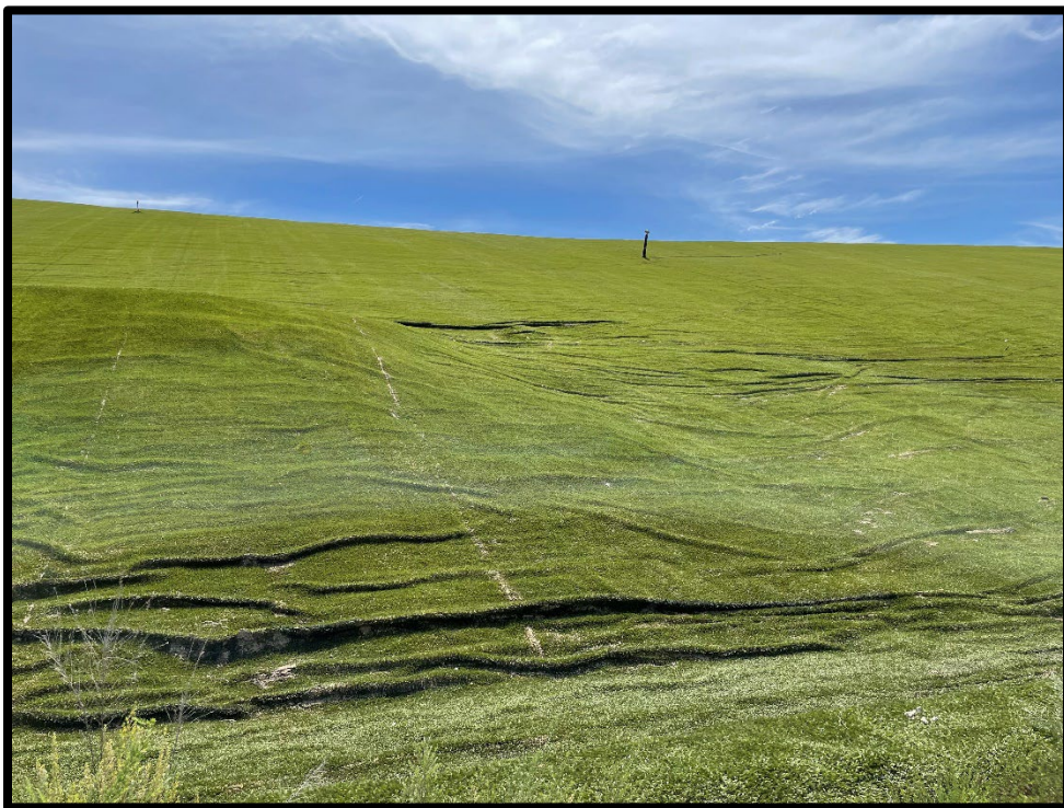
Photograph 8: View of rills present in closure turf of north side of Area 1-2.
