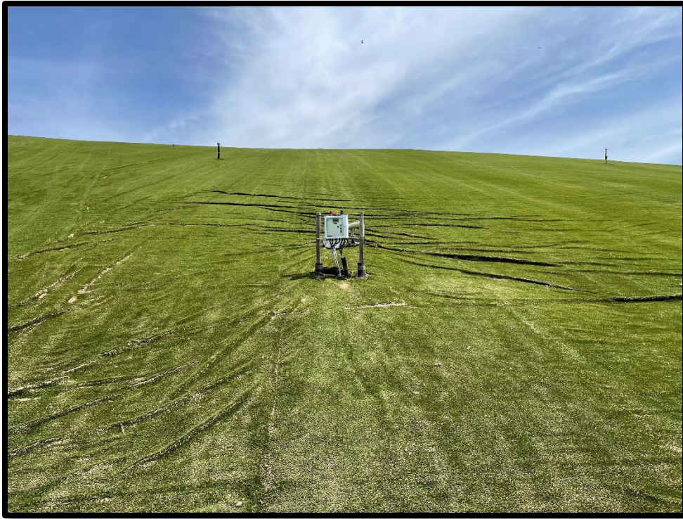
Photograph 9: View of rills present in closure turf near LCS-3.
