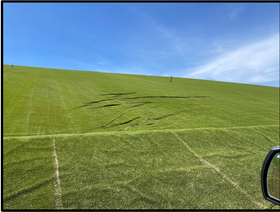
Photograph 7: View of rills present in closure turf of north side of Area 1-2.
