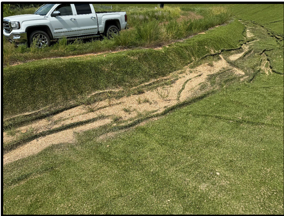
Photograph 16: View of sediment present on closure turf near LCS-4.
