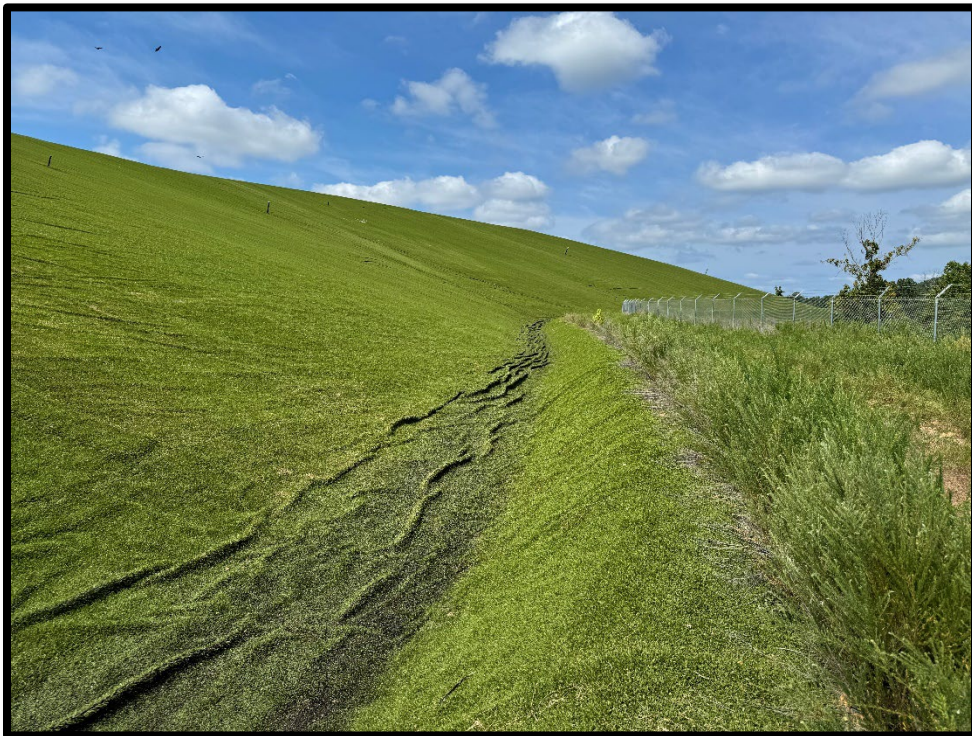
Photograph 4: View of rills present in closure turf of north side of Area 1-2.
