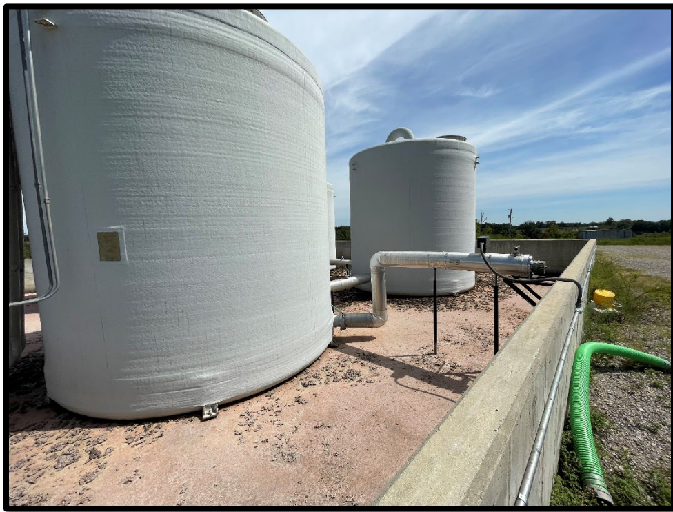
Photograph 2: View of dry leachate tank battery secondary containment.
